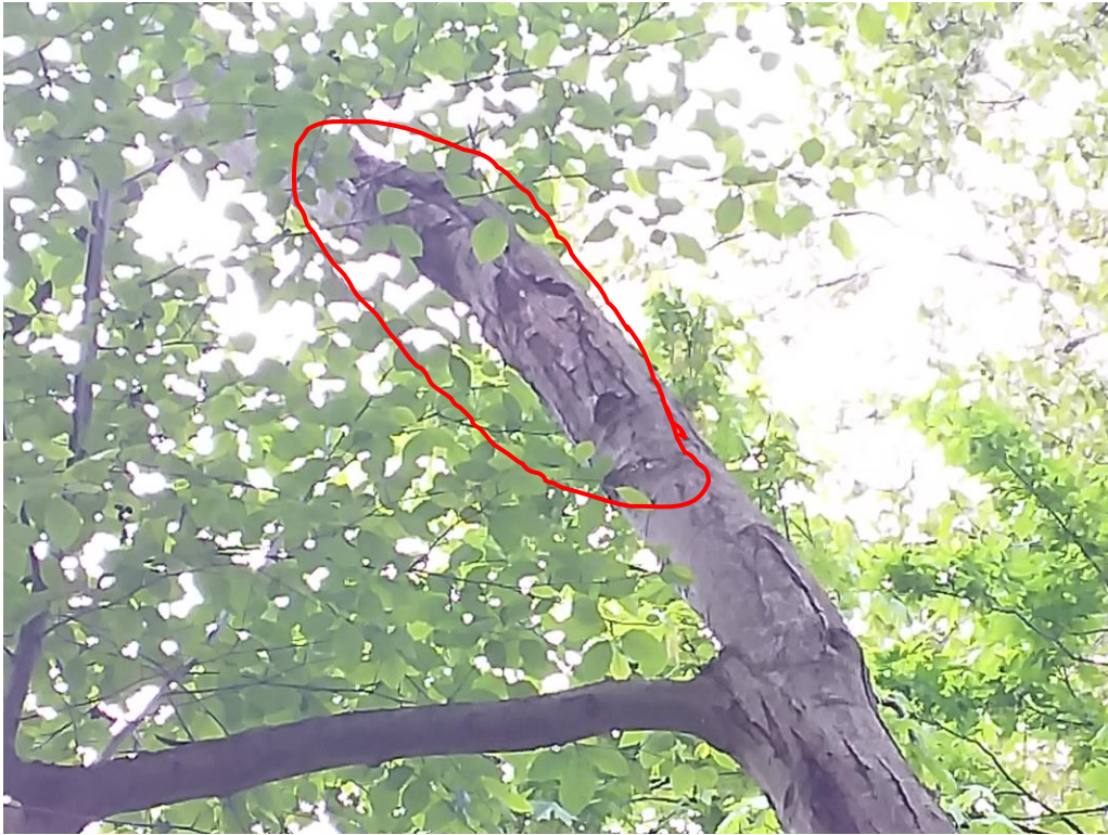
Figure 19. Area of advanced decay in the #21 alder.
